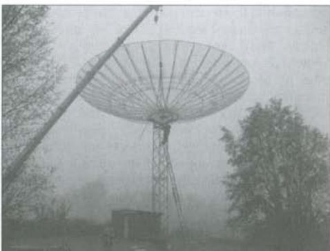
SM4IVE's new 13m homemade 600kg dish, was lifted on the tower on October 21 st , wow! More pictures and video on www.sm4ive.com
